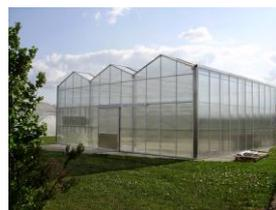
Fig. 3 Prototype on the Venlo type greenhouse of 120m².
