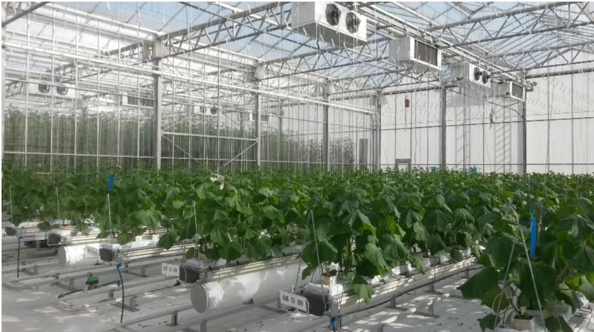
Figure 1. Picture of the greenhouse compartment showing the coolers placed above the canopy below the cover and thermal screen, the growing gutters, the air ducts for dehumidification and the heating transport system
