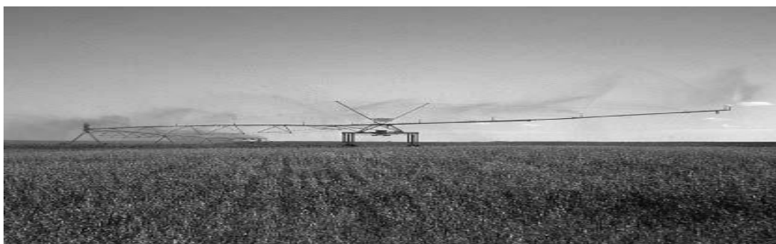
Figure 22 Example of center pivot with corner attachment
