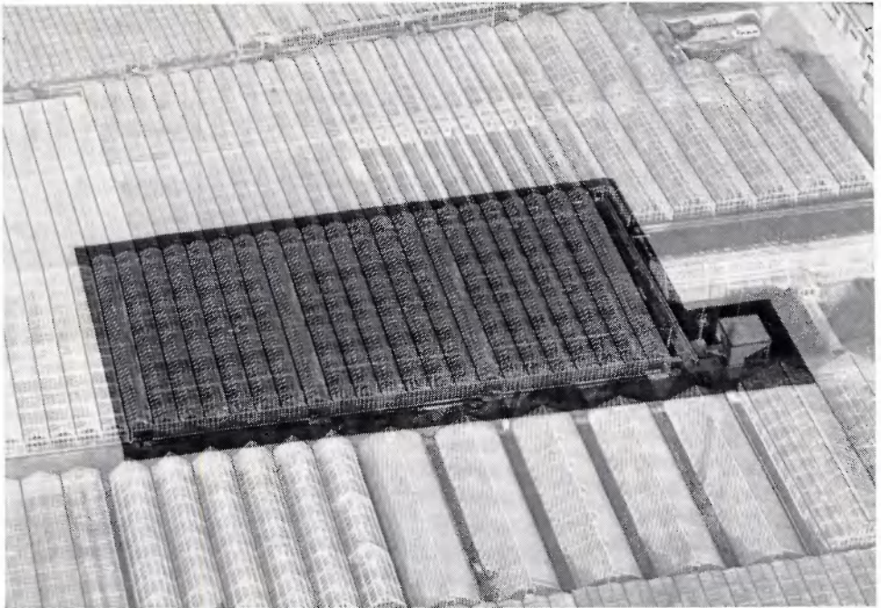
Fig. 2. Aerial view of the climate glasshouse.
