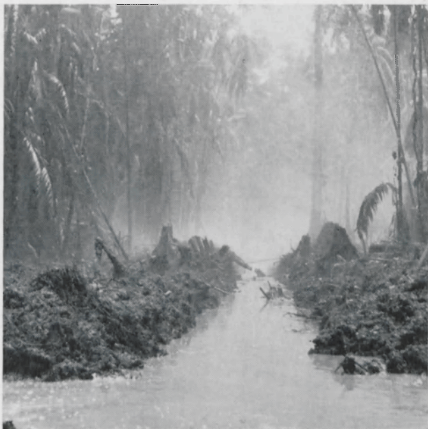
FIG. 10 Results of blasting through clay, in a 10-m wide track, in the perica stand. Trunks and other debris are removed by hand or with portable winches
