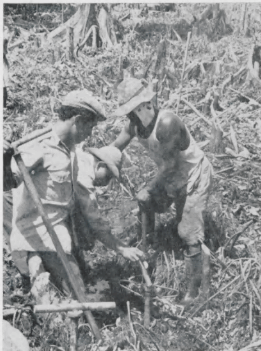
FIG. 6 Punching and loading, one rod being rammed down while the previous one is loaded with sticks of Ditching Dynamite (DD)
