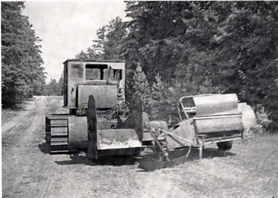
FIG. 4. Equipment for fully mechanized application of layers according to A. T. VAGIN (Minsk, U.S.S.R.). Rear view.
