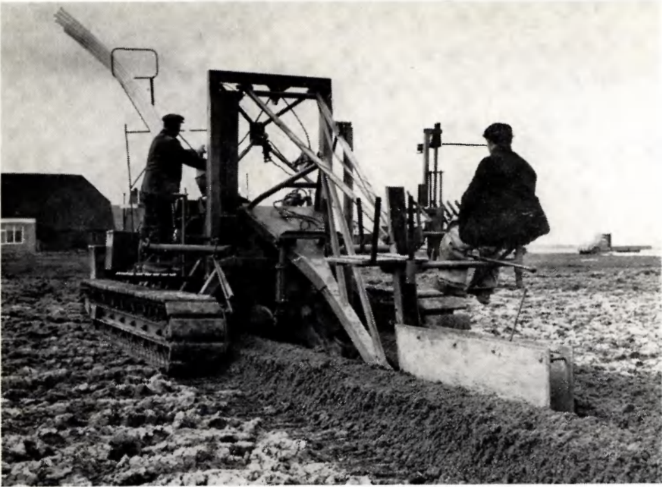
FIG. 4 MACHINE LAYING PLASTIC PIPES.
